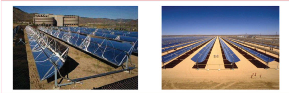
Figure 3. Photographs of two facilities using parabolic trough sensors.
